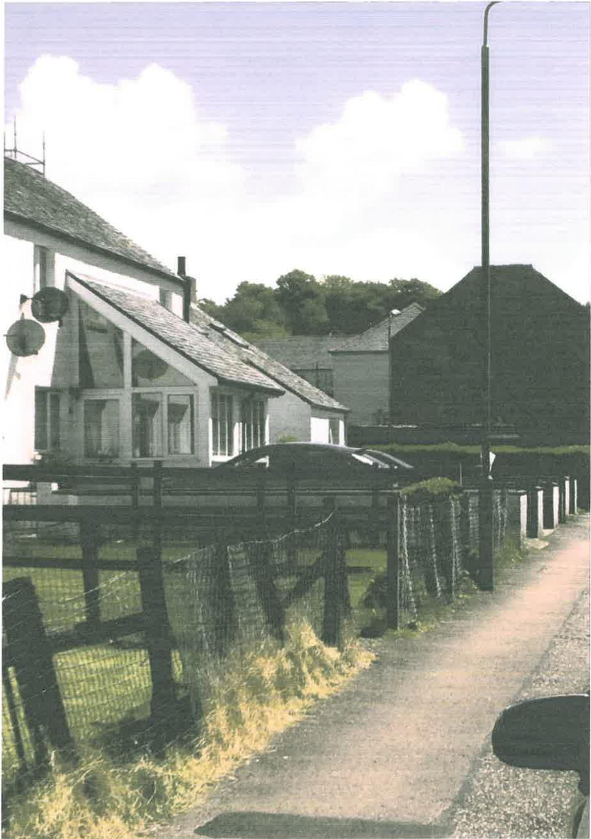
Porch Extensions in Union Street Lochgilphead which are larger than the proposed extension and which clearly overshadow the living room windows.
